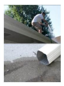
To ensure the free flow of water through the system we suggest running water into the gutter and checking the downspouts for unobstructed water flow.
