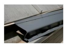
Slide your panel into the slot between the trim coil material and the roofing material.
