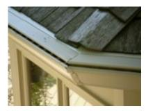
For bay windows repeat the same process, but cut the corners at a 22.5 degree angle instead of at a 45 degree angle.
