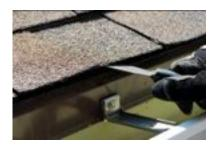
Before beginning the installation, you must determine, based on ease of installation, whether the panels will be best installed under the first row of shingles or between the starter row and the first row of shingles. Use a putty knife to loosen the shingles as needed.
