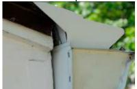
Our end caps are designed to fit six inch gutters without needing to add material. For five inch gutters, hold the end cap up to the end of the gutter and mark as needed to get the proper fitting piece.
