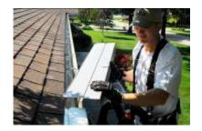
Working left to right; insert the back end of the panel under the shingles. Slide the panel into position on top of the gutter lip.
