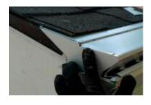
To finish, position the upper flange under the shingles and the installation flange over the cover.
