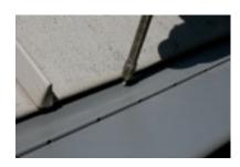
Finally, zip screw the panel to the gutter lip and down through the trim coil.
