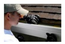
While cleaning, make sure the gutters are properly sloped and sealed.
