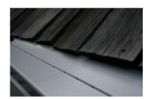
Lift each individual shingle as you slide the rest of the panel into place under the shingles.
