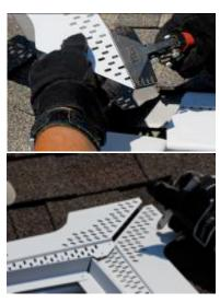
For a closed (or weaved) valley, trimming the miter will easily allow it to slide under the shingle.
