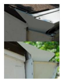
Finally, secure the end cap with two zip screws in the provided pilot holes.
