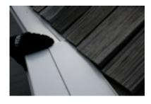
Interlocking the panels on a shake roof can be a challenge. If this is the case, simply overlap the panels to make sure that no gaps are left. If you decide to overlap instead of interlock the panels, use a screw to secure the panels together on the top.
