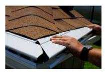
You are ready to position the second panel. Align it with the outside corner, over the top of the tab of the first panel.
