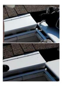
For an open valley, making a few simple bends will allow the miter to better fit the profile of the valley rib.
