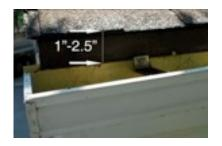
The ideal gutter positioning is 1"-2 1/2" below the roofing material. It may be necessary to raise or lower the gutter. To check this positioning, use a test panel. Ideally, the panel should have a downward slope of between five and twenty degrees.
