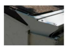
In order to ensure a properly finished end cap there can be no gaps thumb sized or larger.
