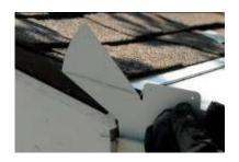
Using tin snips, trim for a tight fit inside the gutter, and mark the upper flange to fit.
